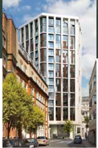
View of refurbished Parker Tower from Parker Street
